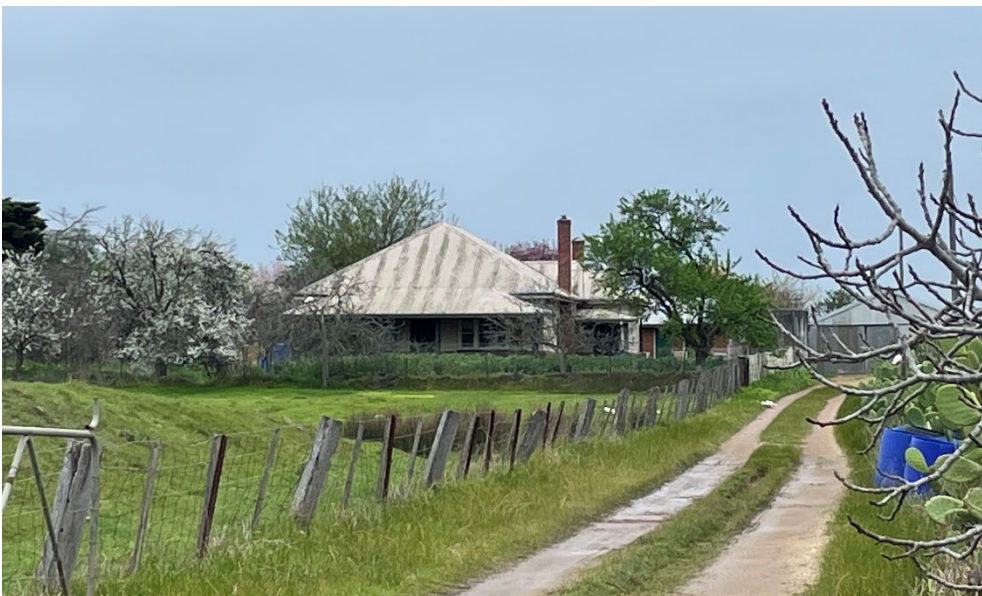
Figure 222 Residence, with steeply pitched roof and chimney visible
