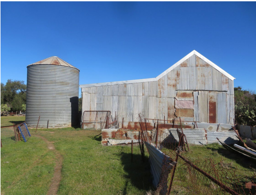
Figure 44 View of farming buildings, including woolshed and grain silo
