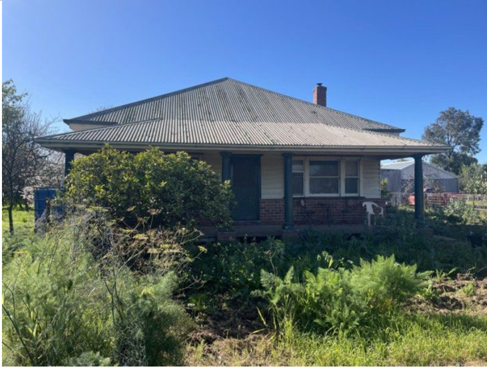
Figure 1 Front (south) elevation of the residence, 80 You Yangs Road, Little River
