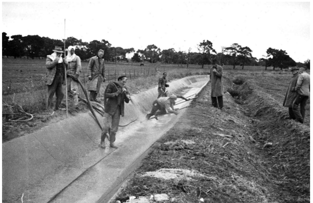
▲ Figure 15. Gunite lining of the 1K channel, Werribee District, c. 1953-54
