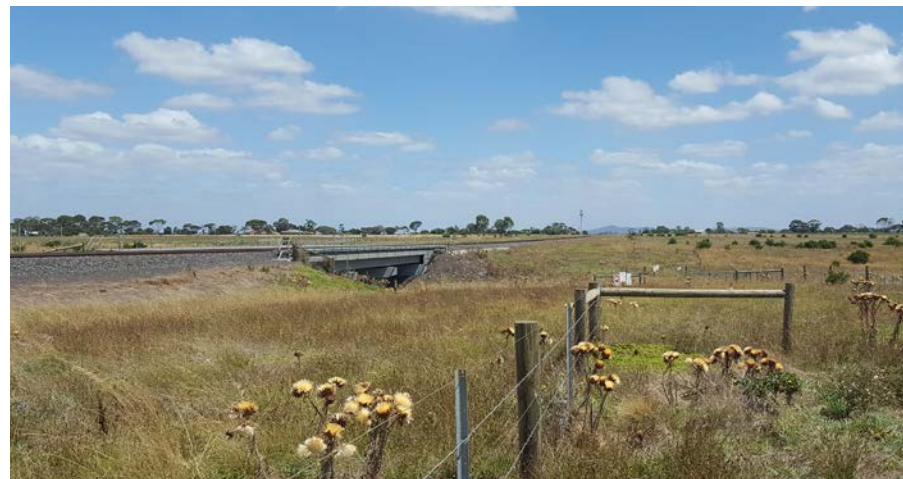
Photo 3 - Train Line Bridge over Davis Creek
