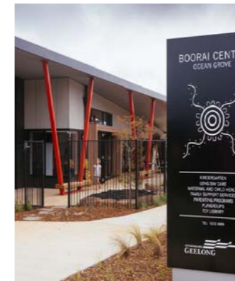
Figure 40: Boorai Centre, Ocean Grove, VIC (Perkins Architects)
