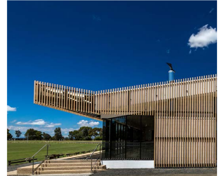
Figure 34: Gordon Street Pavilion, Heyfield, VIC (Katz Architecture)
