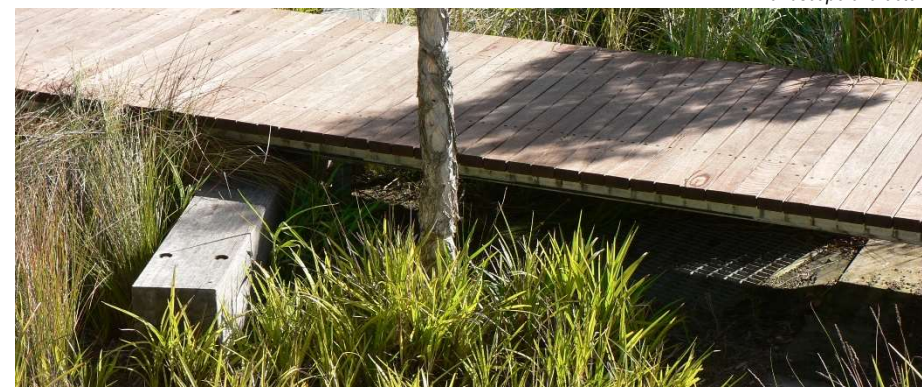
Planted drainage channels
