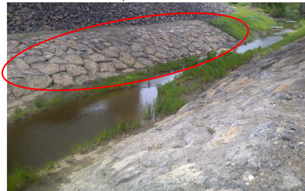
Photo 2: Melbourne Water accepted Armour Stone
