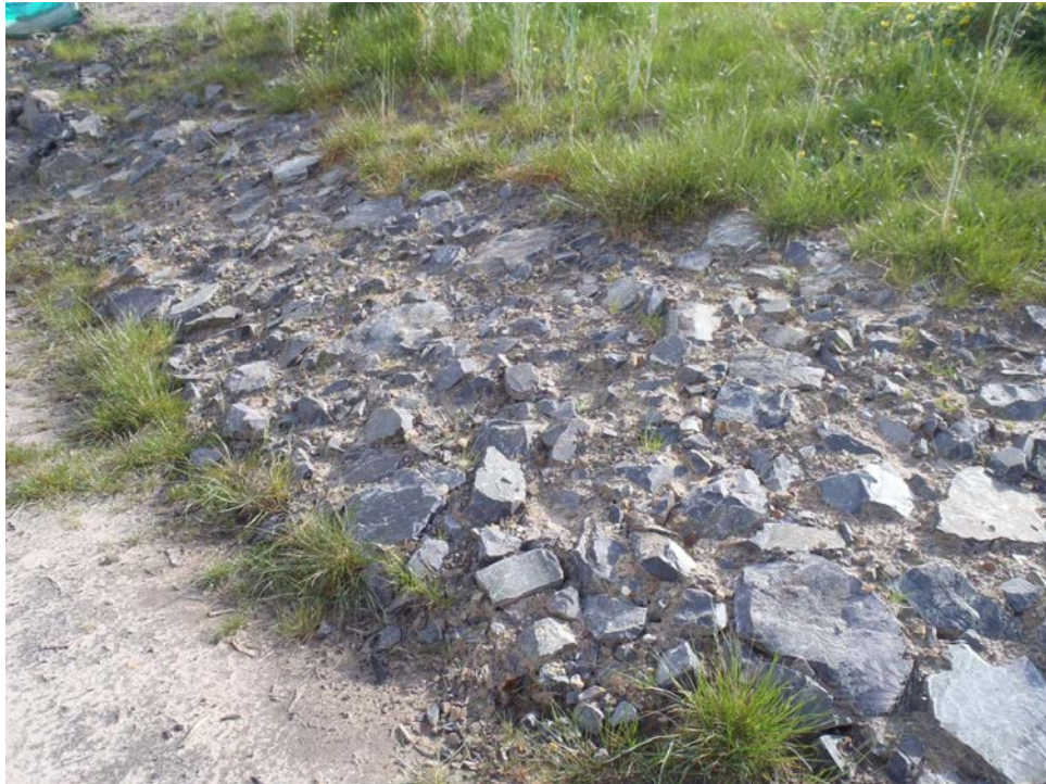
Photo 1: Melbourne Water accepted Type 5 rock beaching
