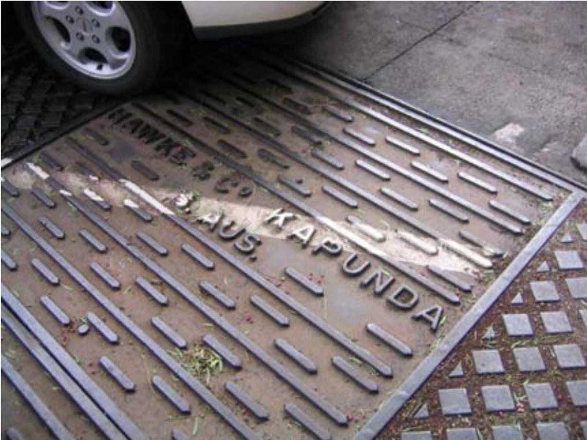
Above: Weighing mechanism in the road surface adjacent to the weighbridge building.
