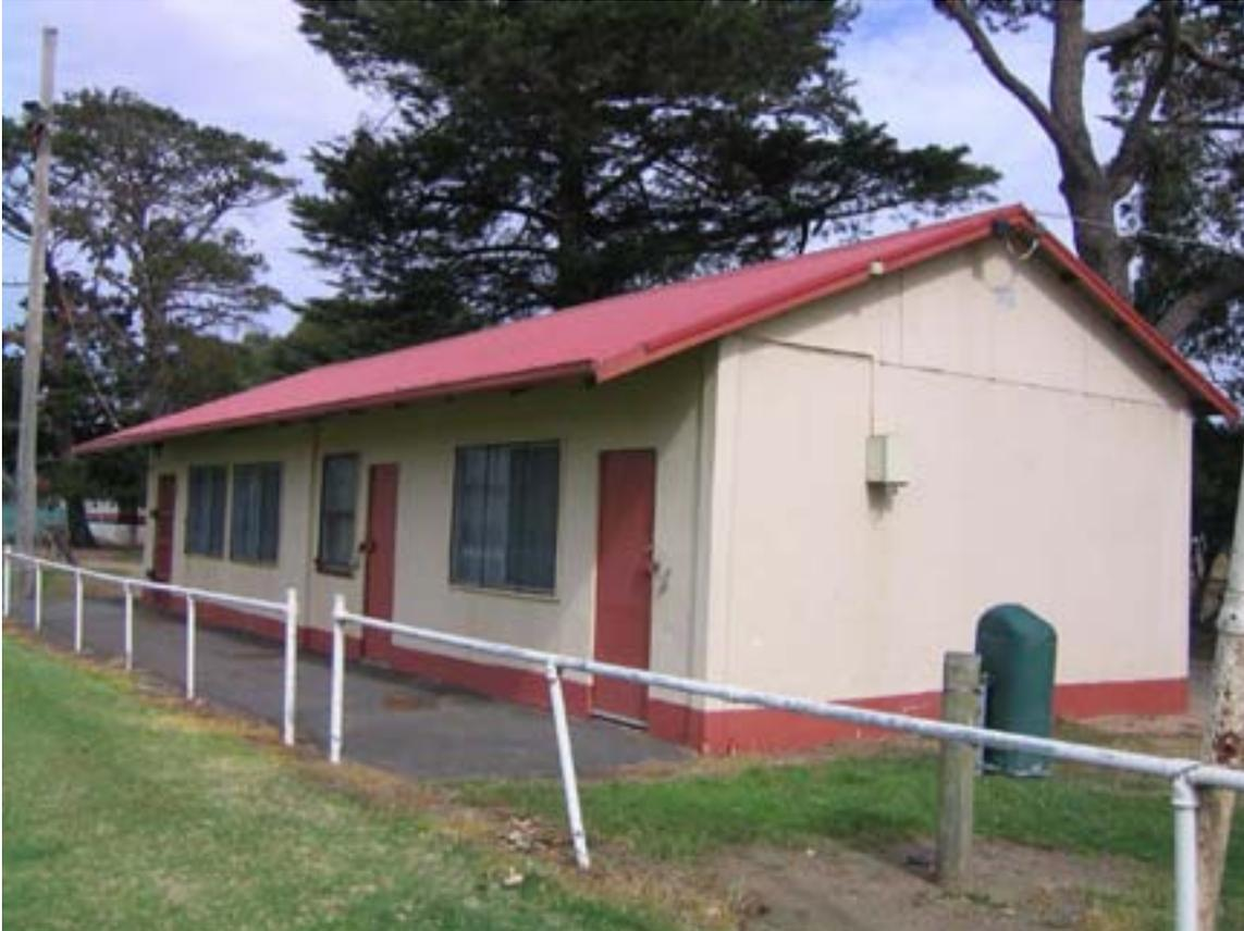
**Above: the concrete pavilion may be made from the precast concrete panel system developed by T W Fowler of Werribee.**
