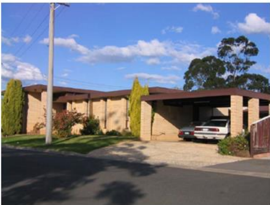
SUMIYA, WERRIBEE (Local significance) TROOPS PARK WEIGHBRIDGE, WERRIBEE (Local significance)
