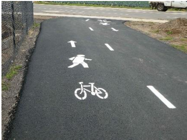
New pavement at Wyndham Harbour has signage indicating to walk/ride on the left. Impressive.
