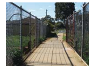
Irrigation channel access bridge
