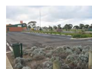
Sealed Car Park associated with Sexton Pavilion
