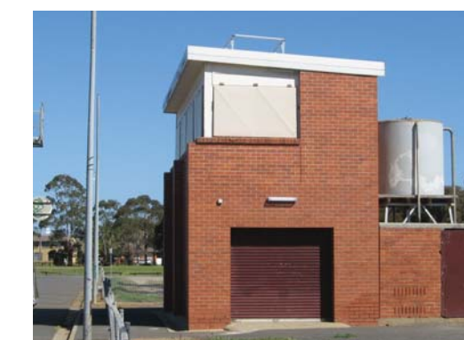
CFA Building and Training Track
