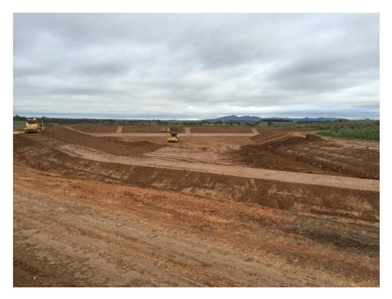
Compacted clay liner currently being installed. HDPE liner installation expected to commence 10 July with practical completion mid August. Commissioning will follow Auditor sign off and EPA approval.
