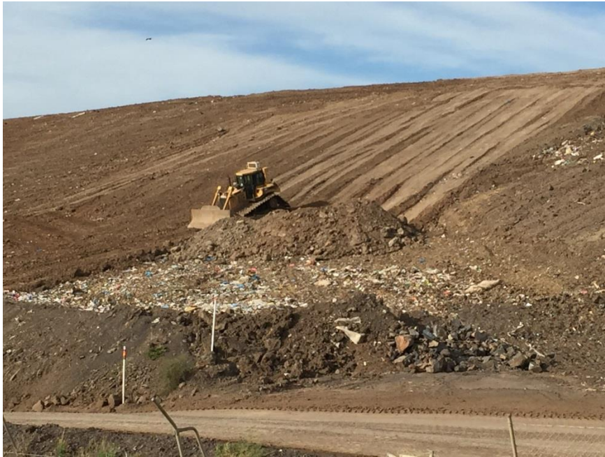
Photograph 5: Placement of intermediate cover, western batters, May 2016
