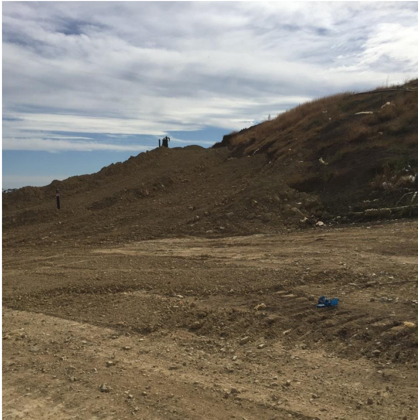
Photograph 9: Placement of intermediate cover around leachate sump on the former Haul Rd - East, November 2016
