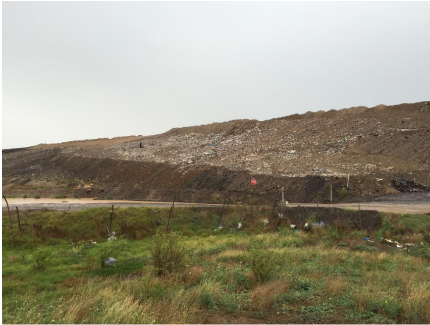
Photograph 3: Filled haul road void space- western batter slope Cell 4A, May 2016
