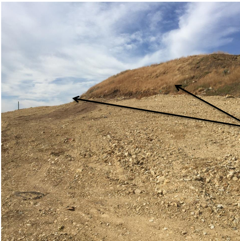
Photograph 10: Placement of intermediate cover around start of the former Haul Rd - West, November 2016 (the areas where additional fill material needs to be placed to achieve 3:1 slope can be clearly seen)
