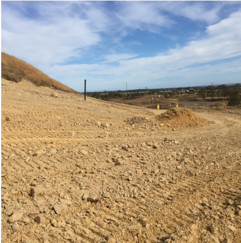
Photograph 11: Placement of intermediate cover around start of the former Haul Rd - West, November 2016
