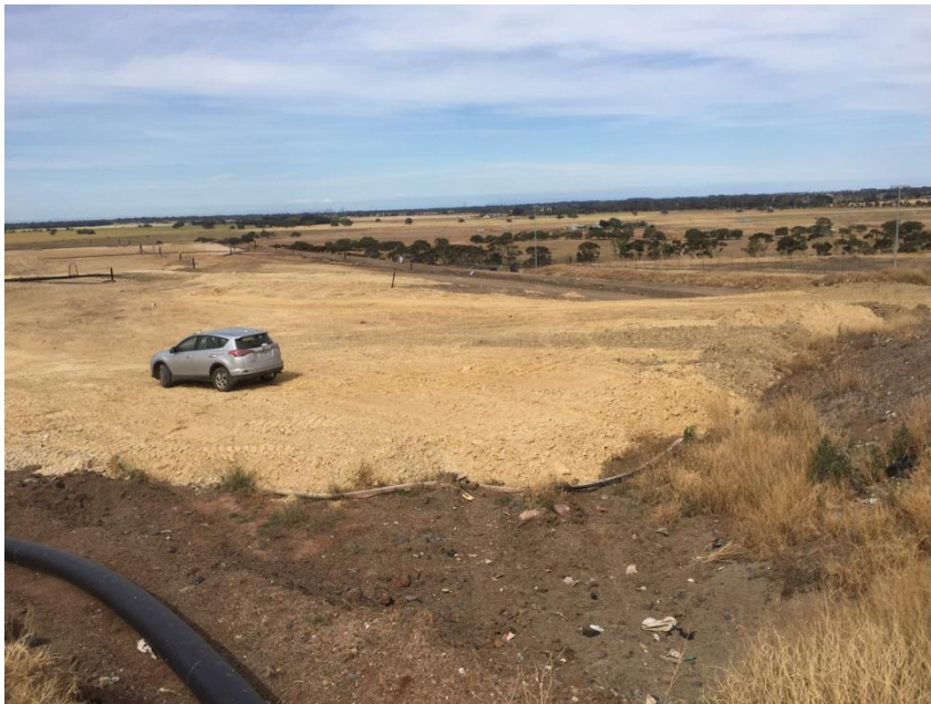
Photograph 8: Completion of intermediate cover, top of Cell 4A, November 2016 (new gas wells on Cell 4B can be seen in the background)
