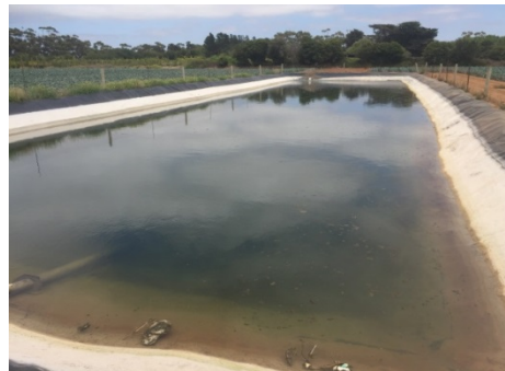
Figure 5: Salt deposits on the sides of a dam in Werribee South
