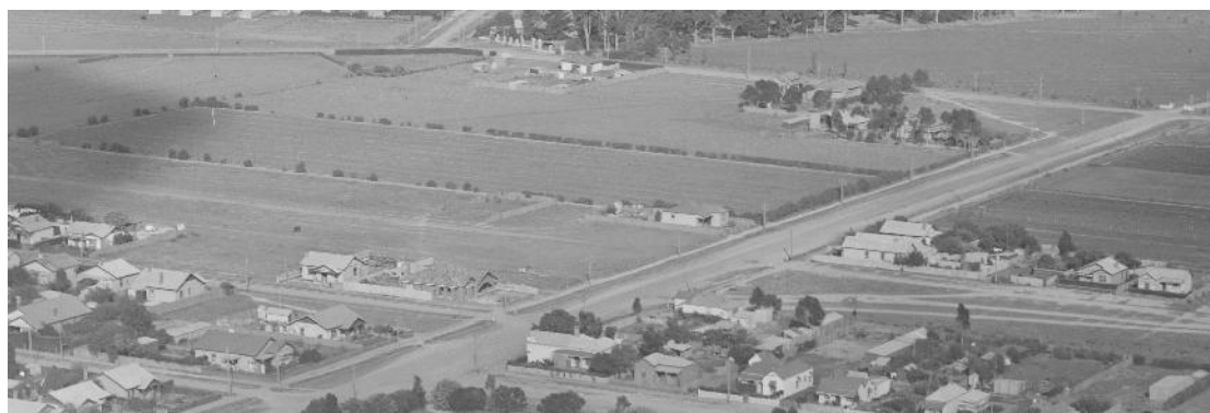
Fig. 2: The land known as Murphy's farm with the line of Bolwell Street in the foreground running left from a new brick house with Wedge Street (the well-made wide road) running lower left to right. In the middle ground is the approximate location of Carter Avenue as yet unformed and occupied by agricultural land. In the rear left is College Road joining Russell Street at the gates to the rear of Werribee Park. (At the time transformed into Corpus Christie College). Source Charles Pratt aerial, State Library of Victoria.
