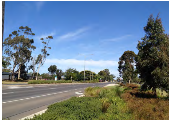
Water Sensitive Urban Design drainage systems
