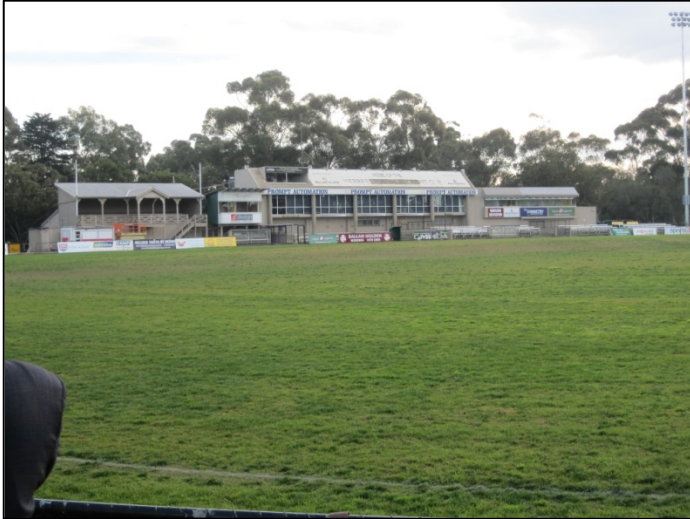
View of Existing Pavilion and Grandstand from South
