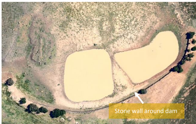
Figure 55: Aerial view of Clarke's Dam Source: Nearmap 2012
