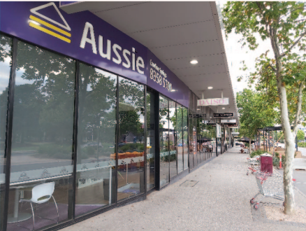
Area 11 - Facade toward Caroline Springs Blvd
