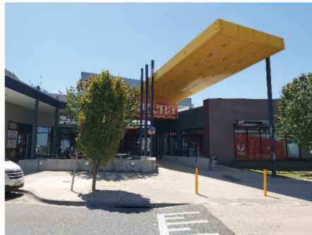
Area 4 - Access from Damon Street
