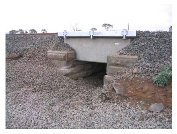
Above: Abutments carrying the railway line over a low narrow culvert 42.92 kilometres from Melbourne.
