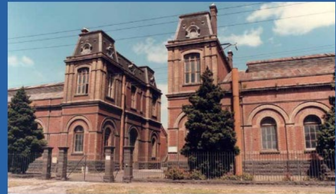
Spotswood Pumping Station
