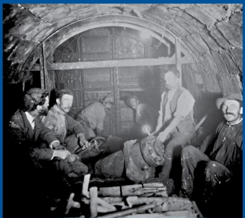
Tunnel shield in compressed air under Port Melbourne. Hobson's Bay Main - 1893
